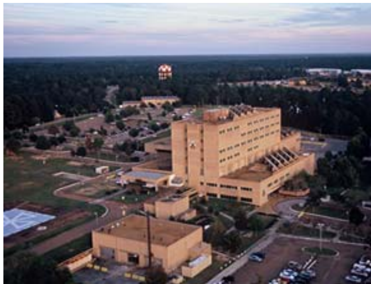
Bayne-Jones Army Community Hospital, Fort Polk
